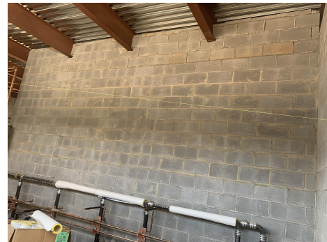
CSK- Concession interior CMU wall installation
